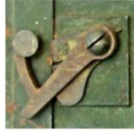
Version 1A, locking swivel catch, fastened by a roundhead screw.
